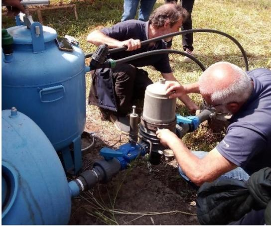
**The technicians Facchin and Saraceno checking the filters of the Ampo Koisha irrigation system**
